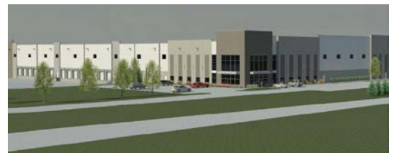
Figure 2: Lone Elm 716, Under Construction
